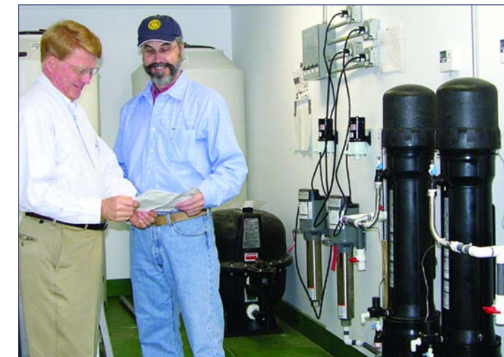
Stan Madsen (left) and Eastern graduate Russ Kehler '78 review the plans for the Nigerian Water Filtration Plant before shipping it to Kwang Village to save lives.
