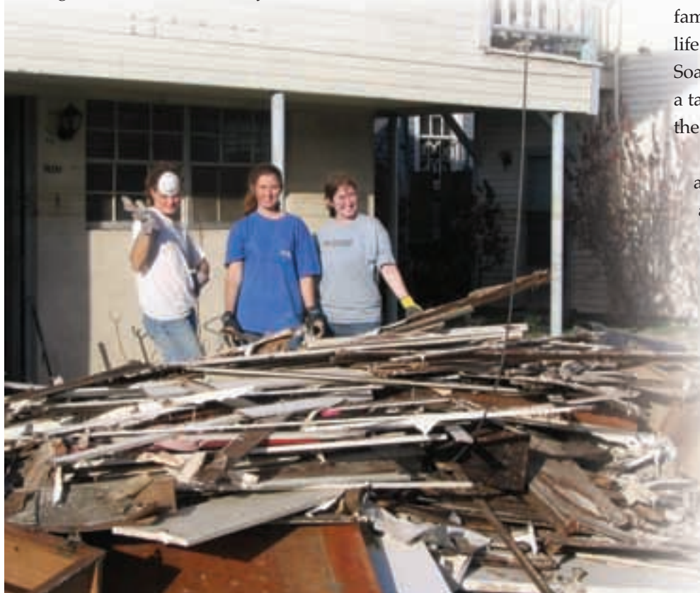
Becca Clyde, (left to right) Catherine Claire and Courtney Darby, standing proudly behind their demolition efforts from the first floor of Richard's home.
