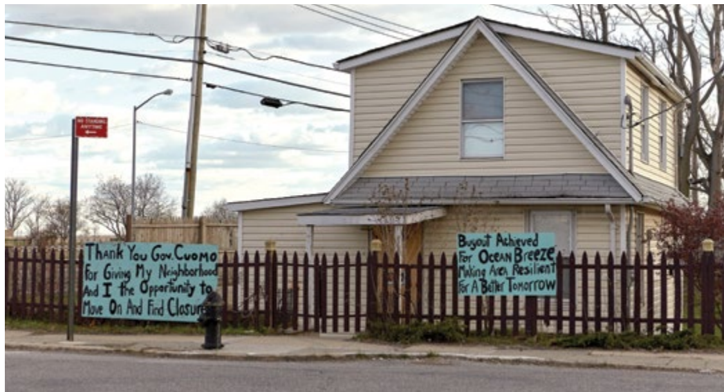
HURRICANE SANDY DEVASTATION IN SOUTH BEACH, ON FATHER CAPODANNO BOULEVARD, STATEN ISLAND, NEW YORK.
